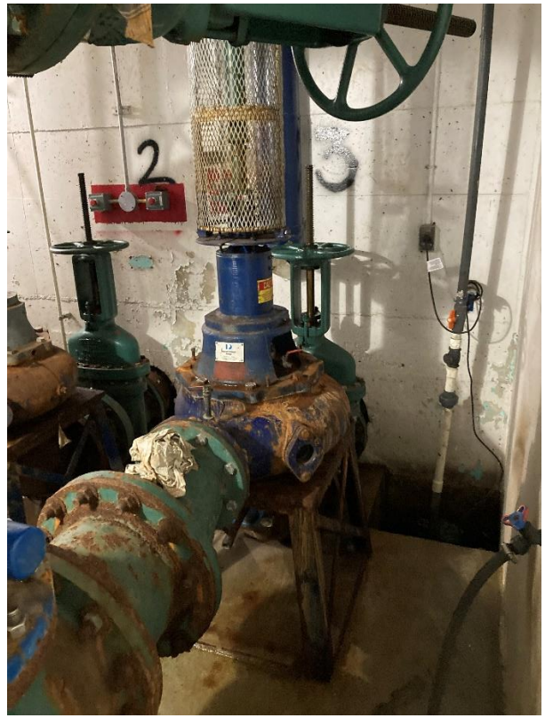
Pump Room – lift pumps and intake piping with gate valves
