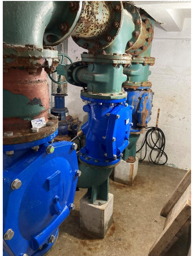
Pump Room – lift pump discharge piping with check valves, gate valves and header
