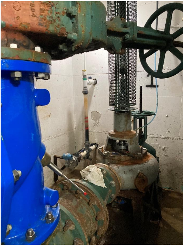
Pump Room – lift pumps and intake piping with gate valves
