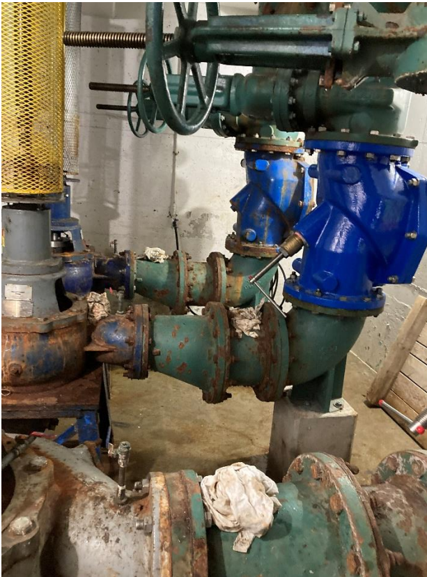
Pump Room – lift pump discharge piping with check valves, gate valves and header
