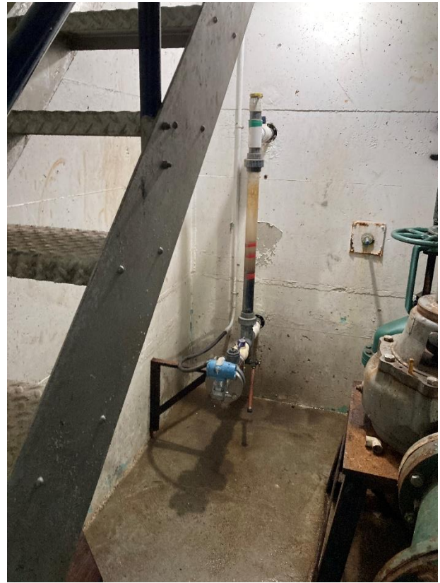
Pump Room – stairs, differential pressure transmitter (for wet well level sensing) and lift pump 1
