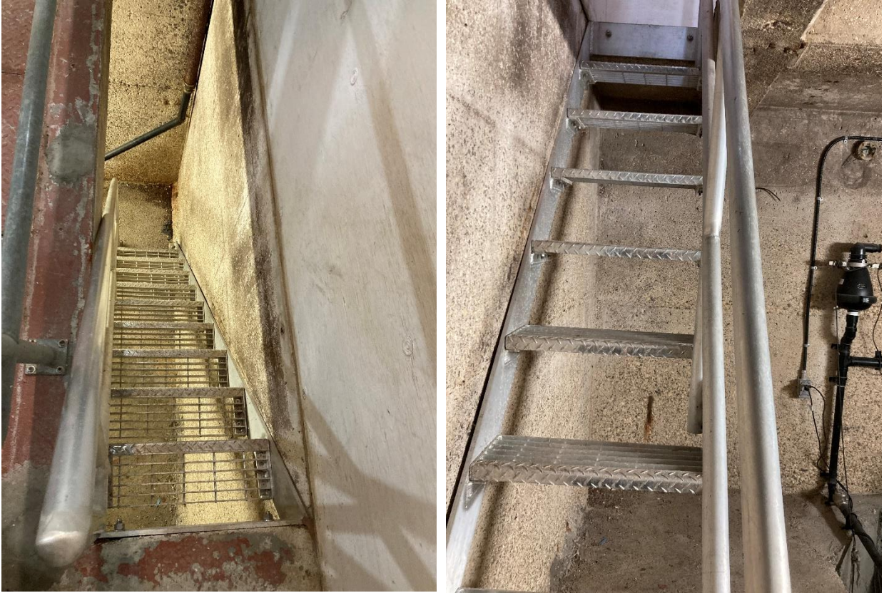
Stairs to Comminutor Chamber
