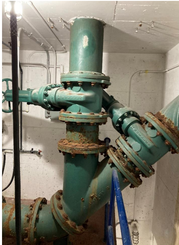
Motor Room – Discharge Pipe to Gate Chamber (vertical) and Force Main (angled pipe)
