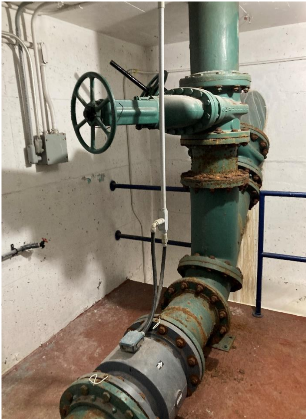
Motor Room – Discharge Pipe to Gate Chamber (vertical) and Force Main (angled pipe)
