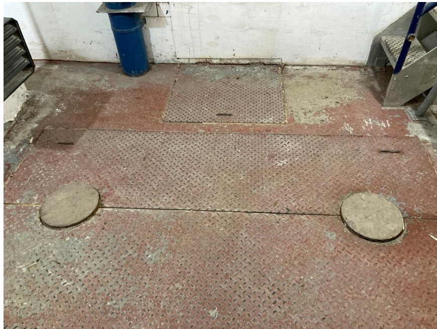
Lower Level – stairs from Main Floor (right), entrance to Motor Room (left)
